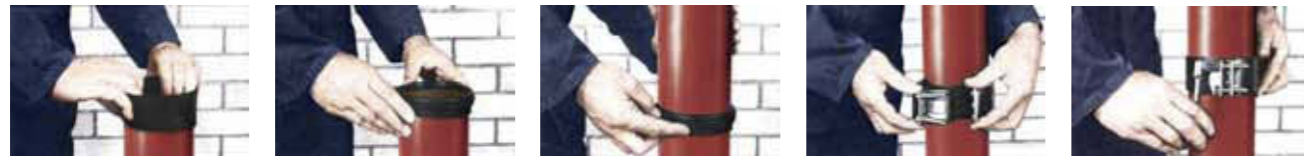
Push the supplied sealing gasket on to the pipe spigot so it abuts the gasket central register
