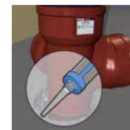
Seal the openings with cement or sealant.
